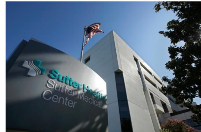
The Sutter Medical Center in Sacramento, part of the vast Sutter Health hospital system in Northern California. Rich Pedroncelli/Associated Press
